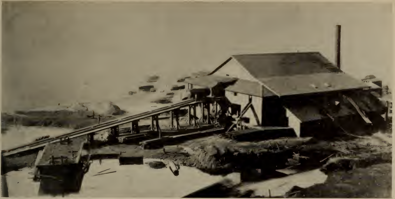
SECOND MILL AT MENDOCINO CITY Built in 1854, mill operated muley saw, two single circular saws with capacity of 60,000 feet a day. (Photo Union Lumber Company Collection)
