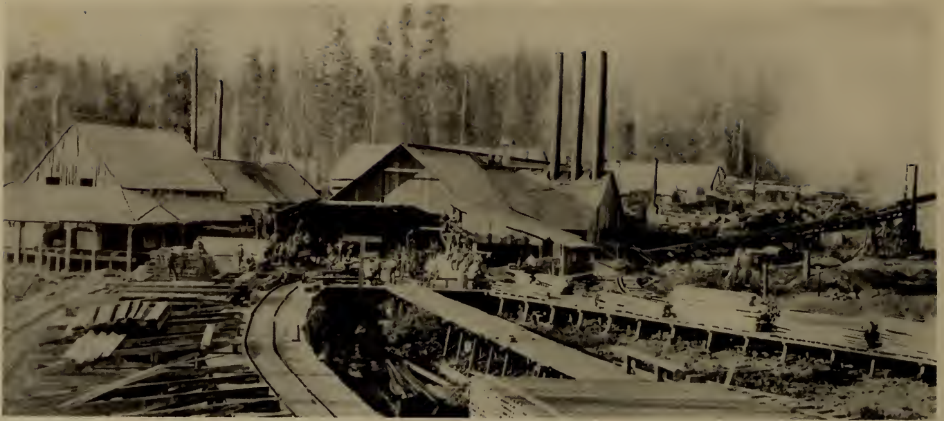
"BIG MILL"—SISSON Original mill on site of present Mt. Shasta Pine Manufacturing Co. First operated in '80s by Bernard, Wallbridge and Huntington, then sold to Leland, Wood and Sheldon. Note wooden tram rails and slab conveyor to open fire. (Photo Kaymore Studio courtesy Siskiyou County Historical Society)
