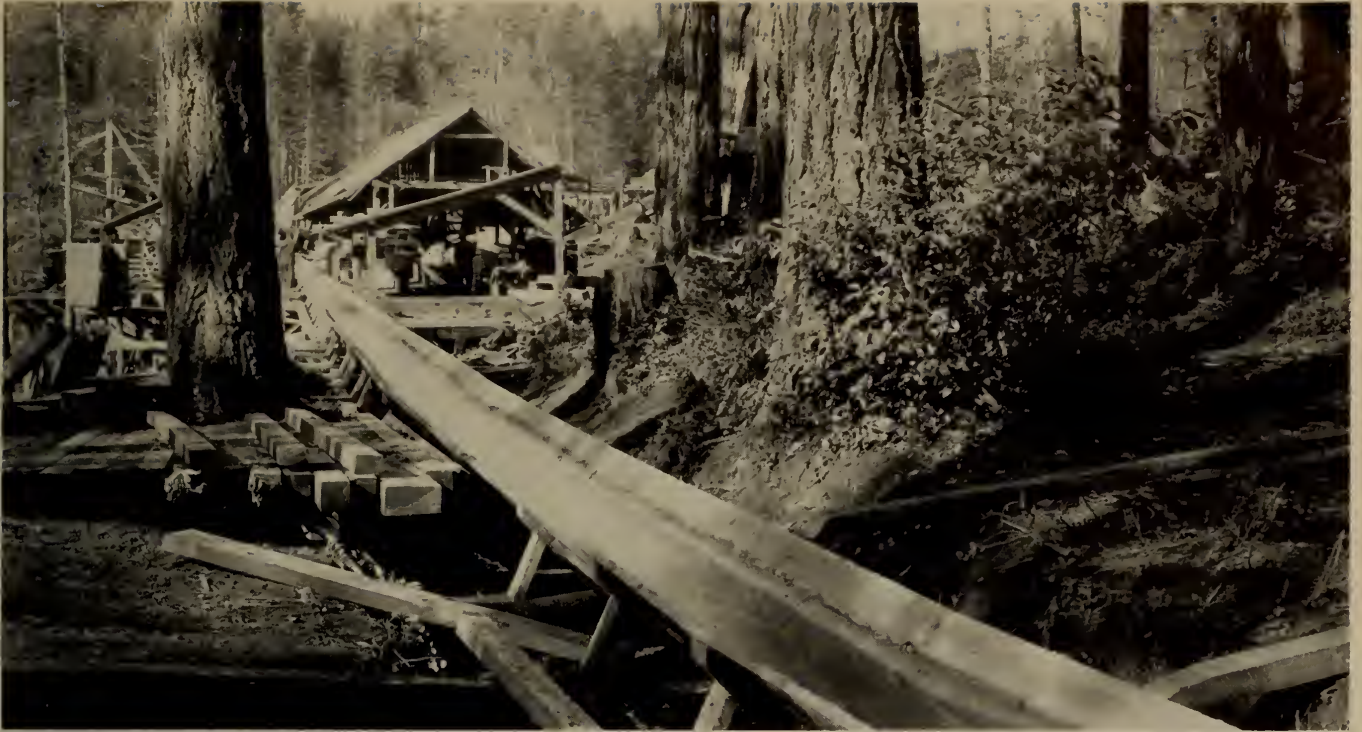
FLUME IN HILLS CREEK AREA. Lewis flume near Dexter, Ore., extended 8 miles from Lost Creek Valley to railside mill at Pengra where it crossed both state highway and middle fork of Willamette River. (Photo University of Oregon)
