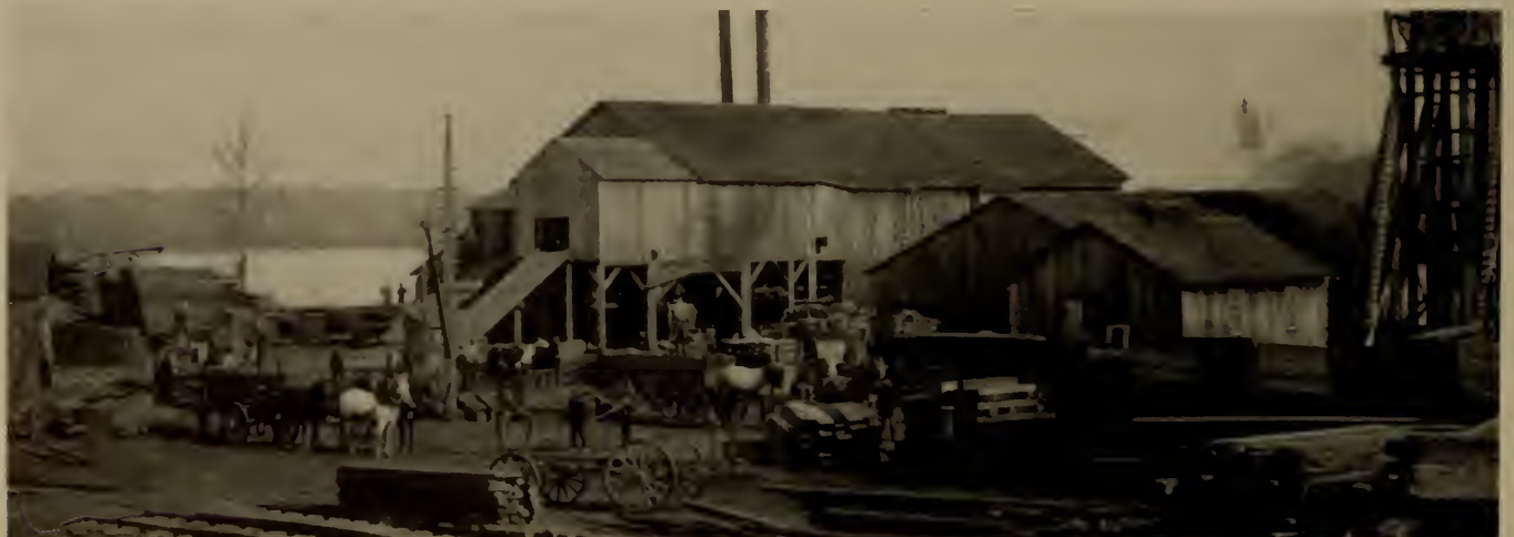
FRONT STREET MILL—PORTLAND about 1905. (Photo Tillamook Pioneer Museum)
