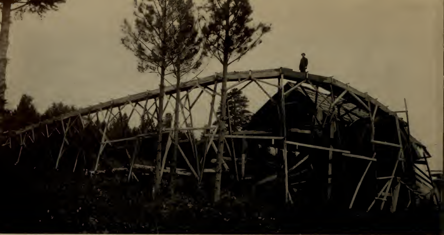
POWER FLUME RAN UP HILL? Camera angle distorts water line of Charles Brown's waterpower mill two miles south of Grangeville, Idaho. (Photo Idaho Historical Society)
