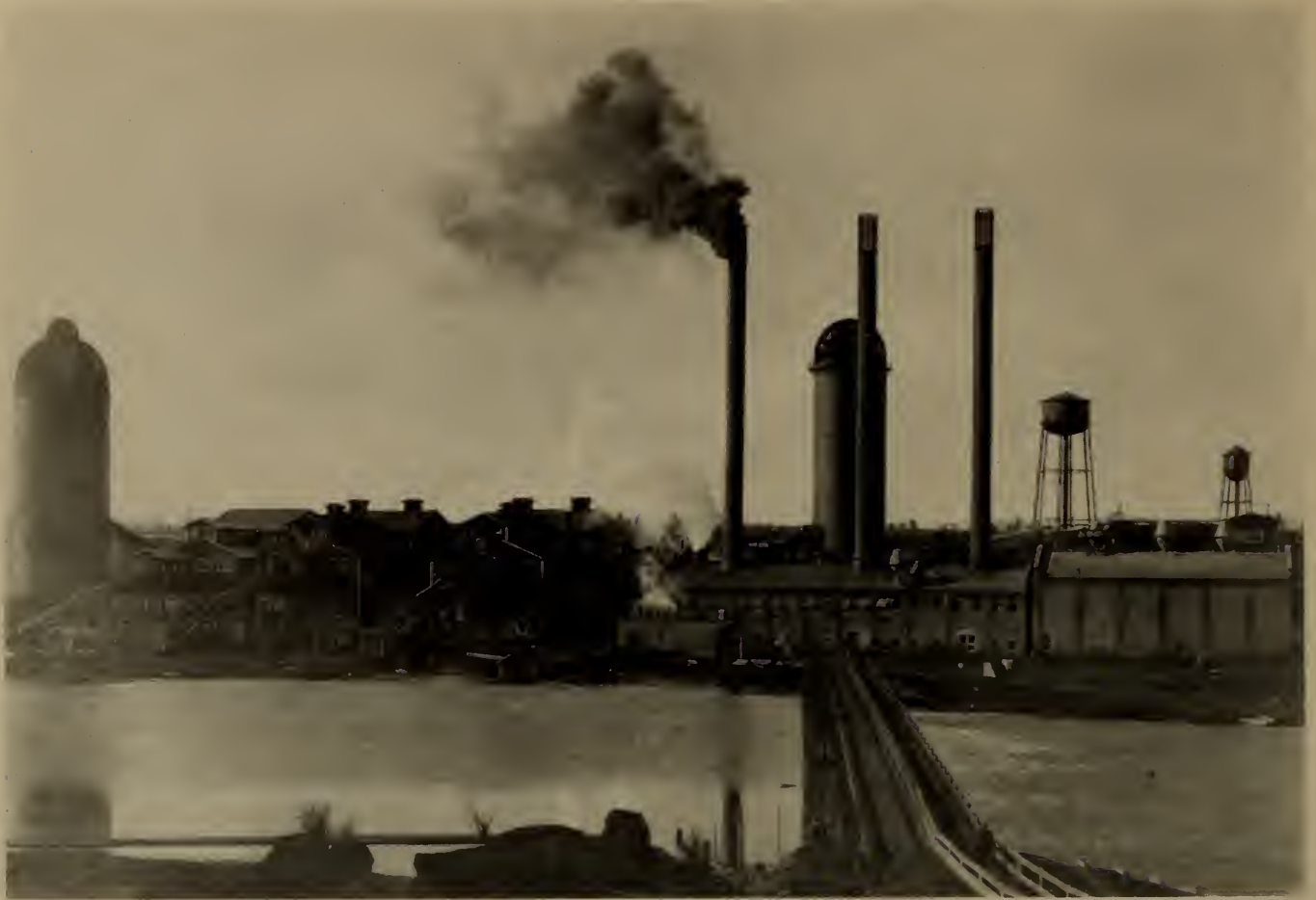
"BURNER COST A MILLION" — it was said in Bend. Big Shevlin-Hixon Lumber Co. mill in Bend, Oregon, with its three stacks and log slips. Burner on the left was over 100 feet high, built of fire brick 4 feet thick and covered with \frac{1}{2} and \frac{3}{8} inch steel plate. When mill was abandoned, burner was scientifically dynamited, steel sold to sheep ranchers for use as water tanks. (Photo by Ray Van Vleet)
