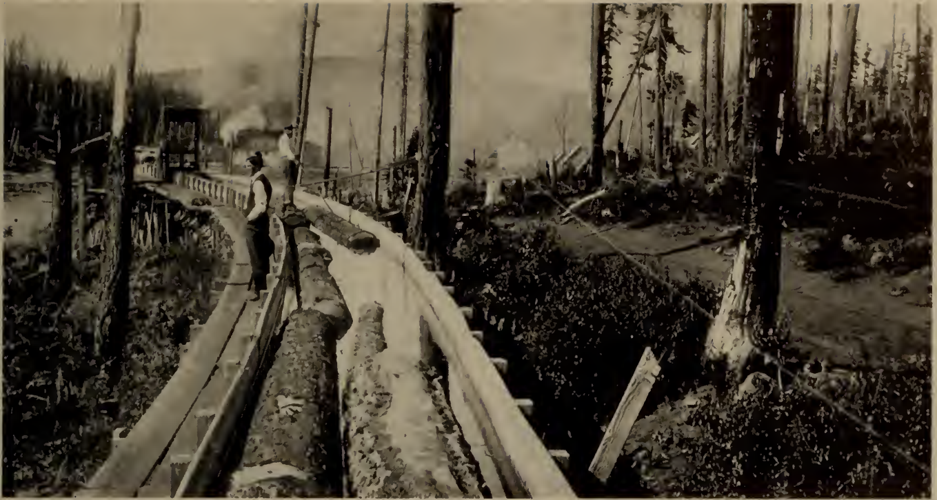
1800 FEET DOWN TO COLUMBIA GORGE went the Bridal Veil flume carrying "a billion board feet in half a century." Trestles were 100 feet high in some places, the trough 4 feet wide at top, handling stock up to 12"x12"x40'. (Photo University of Oregon)
