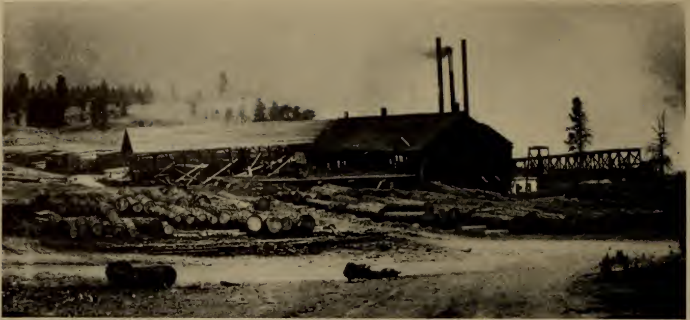
FREE CIGARS WHEN CUT WAS 40 THOUSAND Collier mill at Swan Lake near Klamath Falls, Ore., in 1921. "This was some mill," says A. D. Collier. "Logs came in mill on rollway and tram cars. We usually got about 35 thousand feet in 9 hours with 50" top and 44" bottom saw, 2-block carriage with screw feed and hand setworks. When we hit 40 thousand all hands got free cigars. We had water buckets on the roof and open fires in the slab pit. This was sawmilling!" (Photo Collier Collection Collier State Park Logging Museum)
