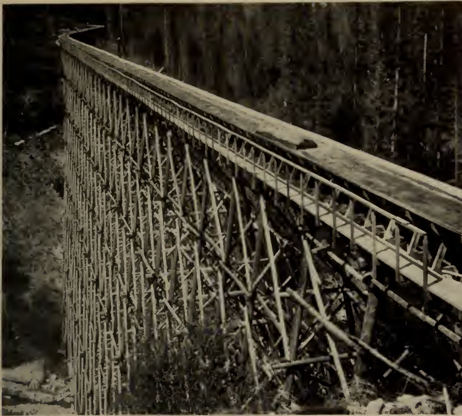
53 FLUMES IN BRITISH COLUMBIA This Bear Creek line at Adams River, Chase, B.C., was one of the largest. They ranged from a few hundred yards long to the 22 mile flume on the upper Moyie River which bored 300 feet into a mountain. (Photo British Columbia Provincial Archives)
