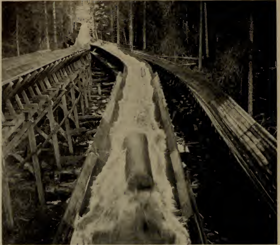
3-WAY FLUME AT BENEWAH CREEK in St. Joe National Forest, Idaho. Each line went to a different point and water was diverted as need occurred. Some Idaho flumes had grades up to 12 and 15%. (Photo William Roddy courtesy Chas. H. Scribner)
