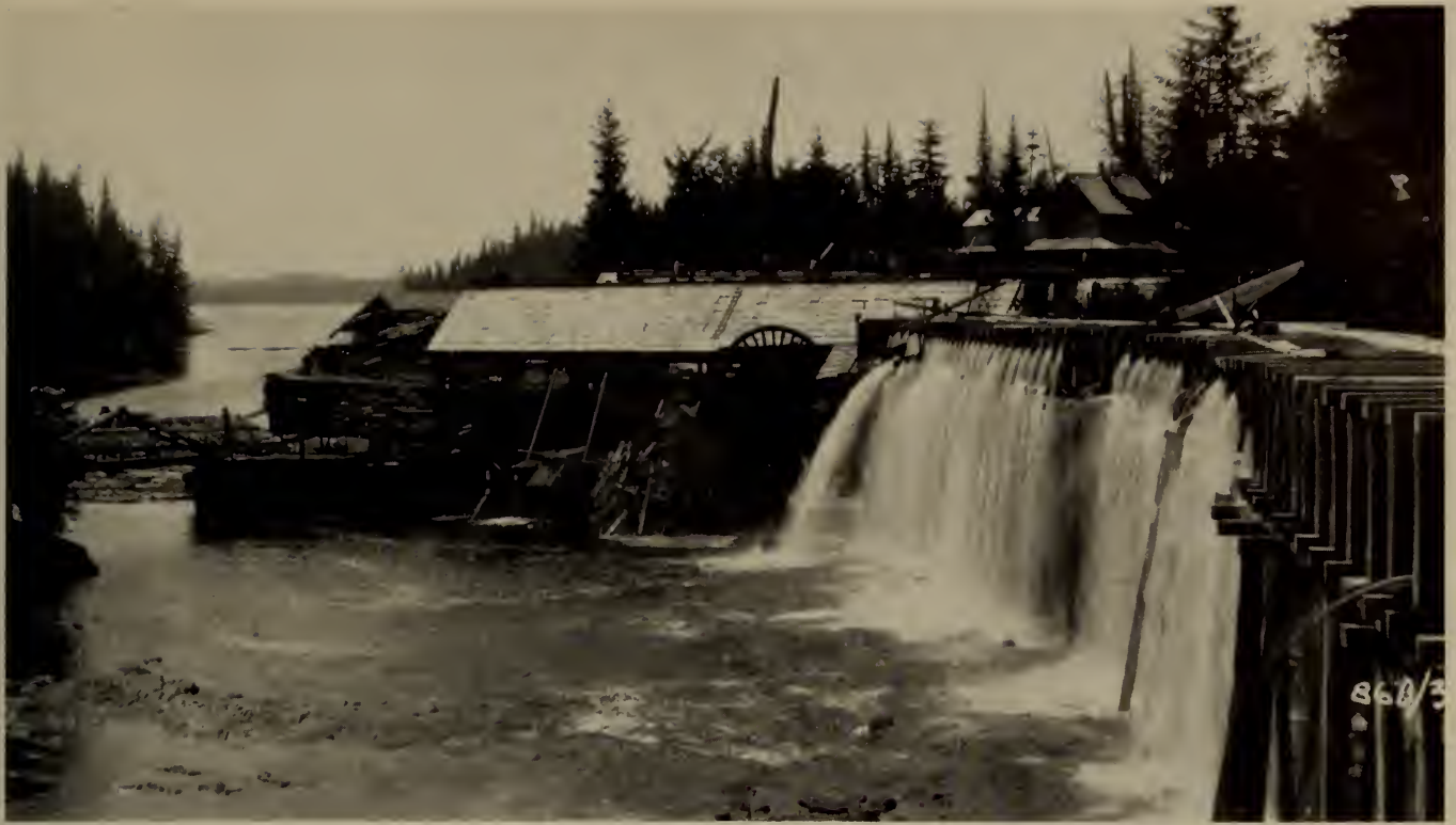
OLDEST SAWMILL IN NORTHERN B.C. Famous Georgetown mill built of hewn timber by George Williscroft in 1875 on Big Bay, 17 miles north of Prince Rupert. Water wheel was used for power at first giving an output of 5000 feet a day. Mill was improved and after George Williscroft's death in 1895, operated by his brother W. A. Williscroft and several other succeeding companies including Big Bay Lumber Company. (Photo British Columbia Forest Service)
