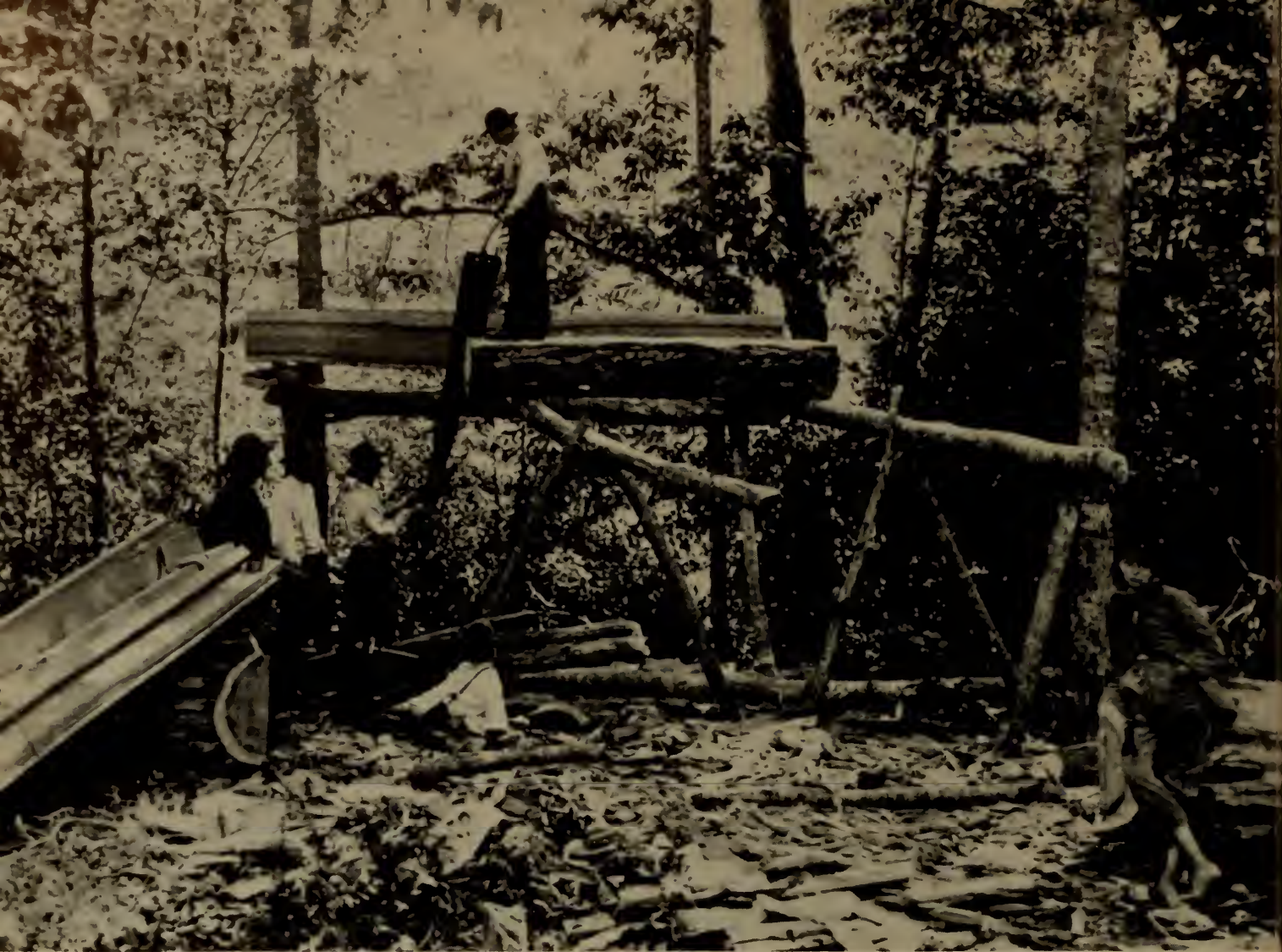
THEY DID IT THE HARD WAY Whip or pit sawing before the turn of the century. Saw was pulled and pushed by men above and below pole trestle. The big trick was to get the log on the platform. This method was used in California in the '80s and '90s, in Alaska as late as 1905. (U.S. Forest Service photo from W. C. Lumbermen's Association)
