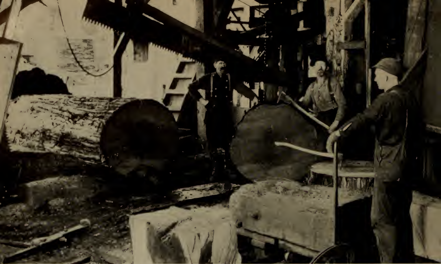
GRAYS HARBOR SHINGLE MILL Interior of Aloha Lumber Co. mill at Aloha, Washington. Logs were sawed, cut into blocks and passed to equalizer at right. (Photo University of Washington)
