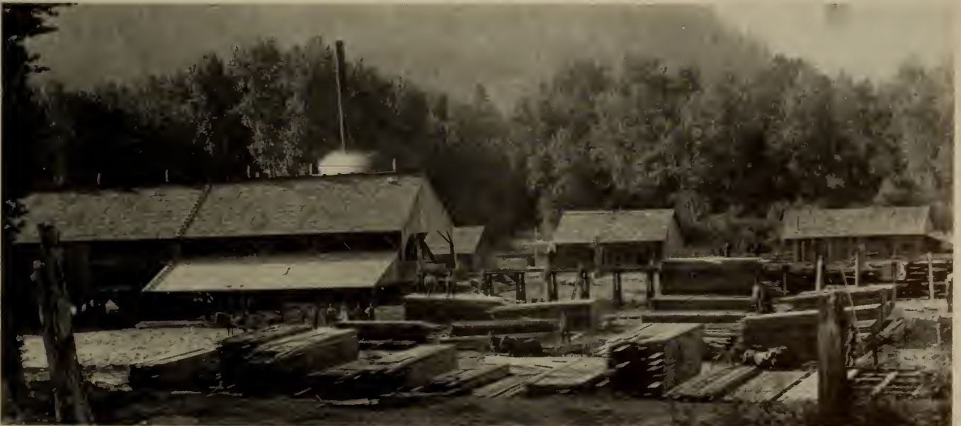
EARLY IDAHO MILL at Cataldo. Ladders ran up roof to water barrels which were of little avail when forest fire raged and destroyed mill. (Photo Idaho Historical Society)
