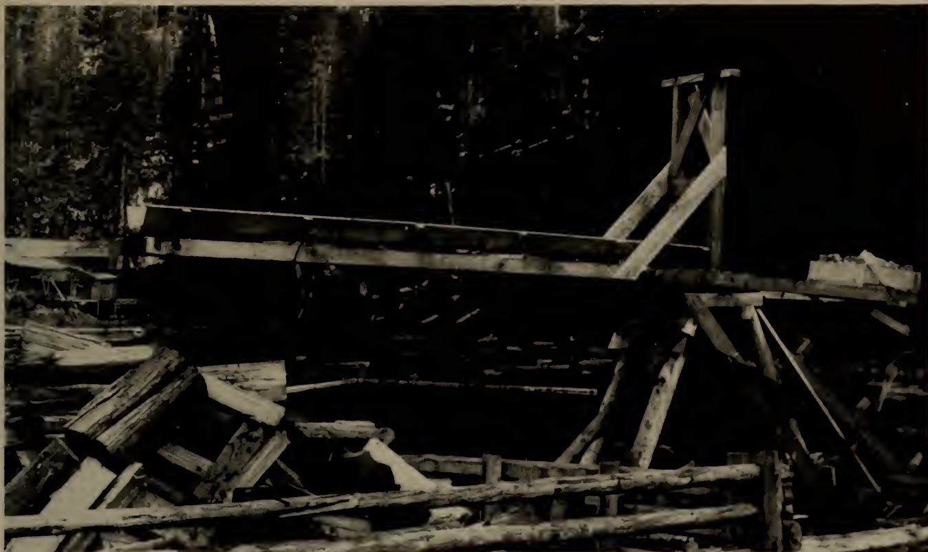
SHINGLE BOLT LOADING RIG in 1925 driven by gasoline engine. Chain belt picked up bolts from pond, dumped them in crib. (Photo courtesy British Columbia Forest Service)
