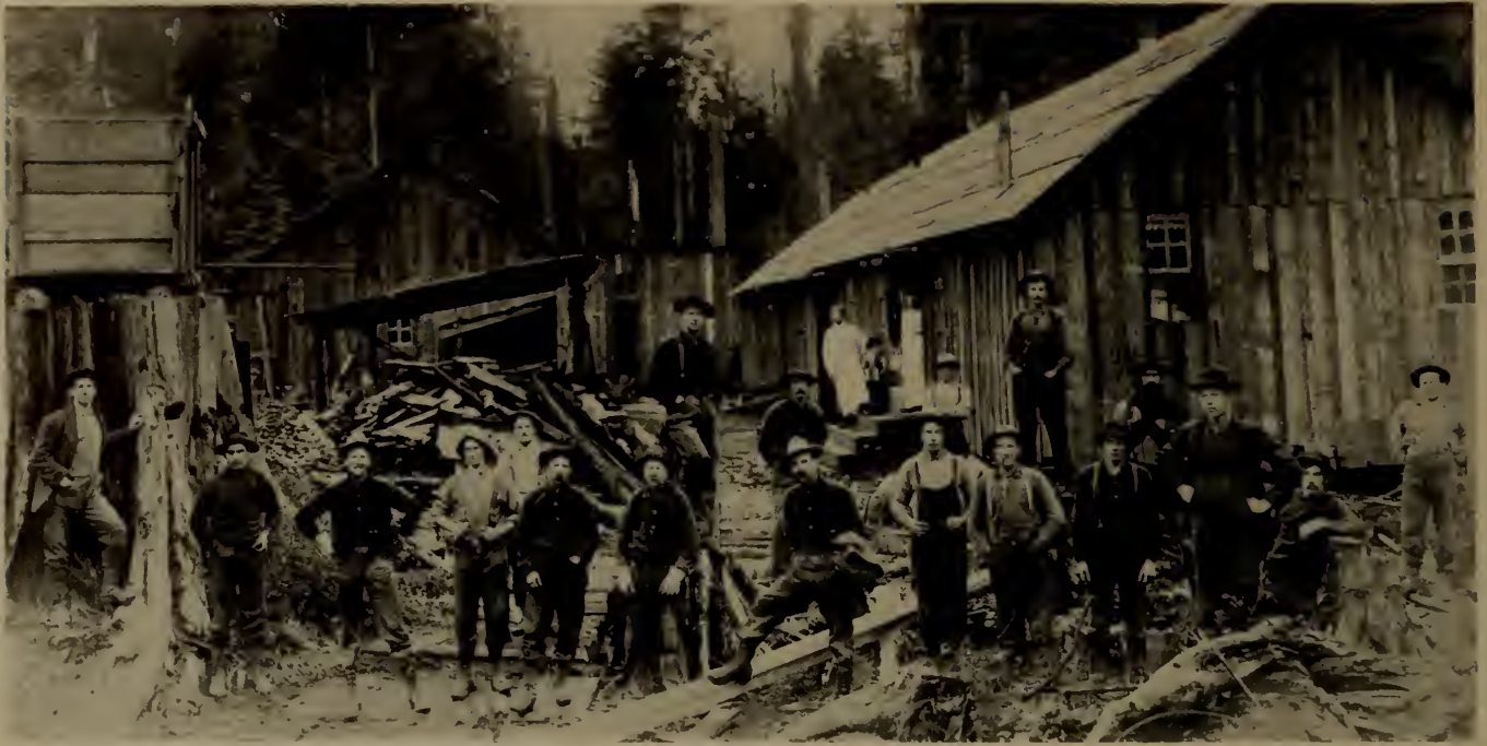
COOKHOUSE AT ROBE —Best Shingle Co. This was known as the Tunnel 2 Mill and was operated by Frank Davis near Robe, Wash., from 1906 to 1910. (Darius Kinsey photo courtesy Ray Moore)
