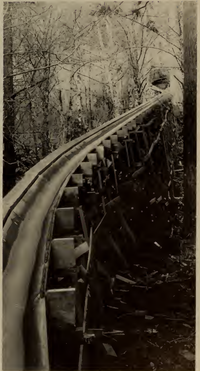
OREGON LOG FLUMES held out over trucks a long time. The Pengra line was built by enterprising Eugene business men. Northeast of Eugene several flumes ran down to Mariola. Southern Pacific flumed from three big mills, Fischer Lumber Co., 6 miles from Parsons Creek. (Photo University of Oregon)
