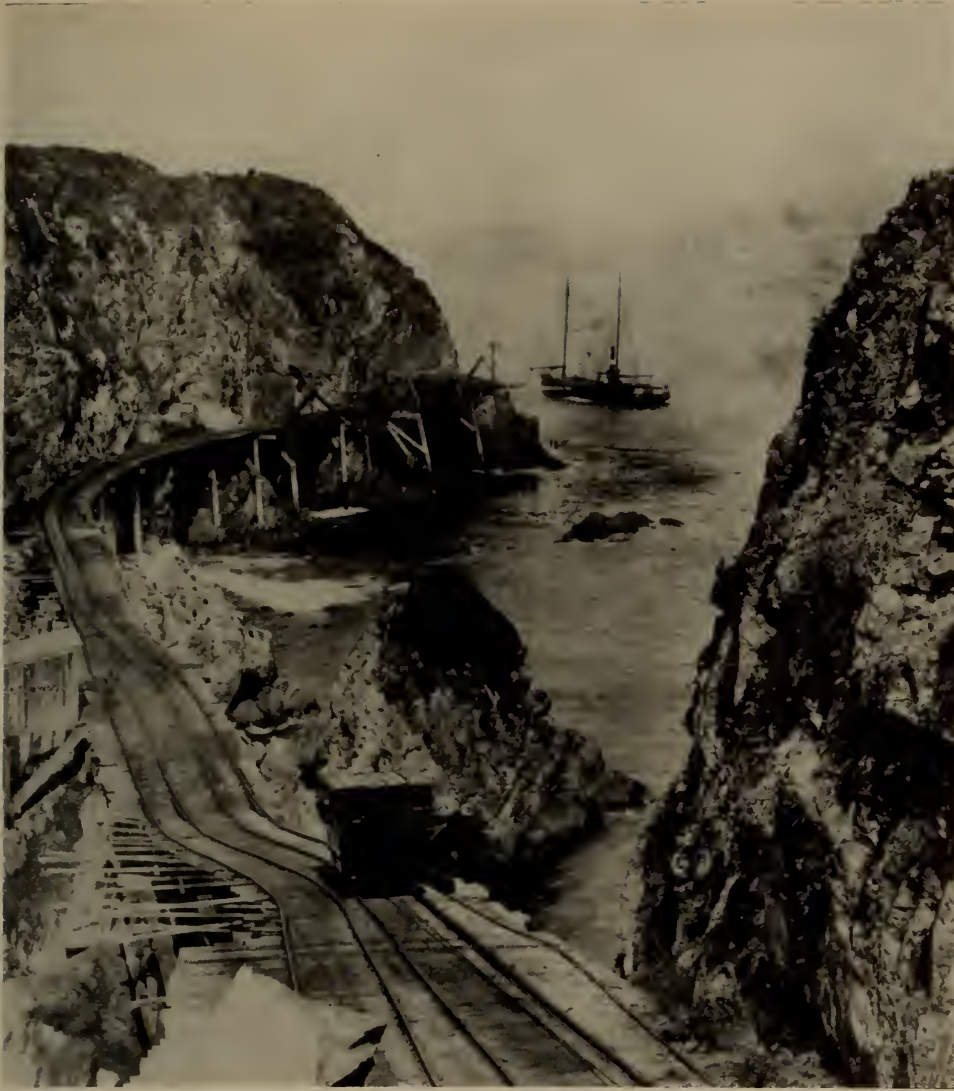
INCLINE TO SCHOONER Redwood lumber at Greenwood Creek was lowered down this narrow gauge incline and loaded on ships by chute. Schooner is Whitesboro. (Photo Union Lumber Company Collection)
