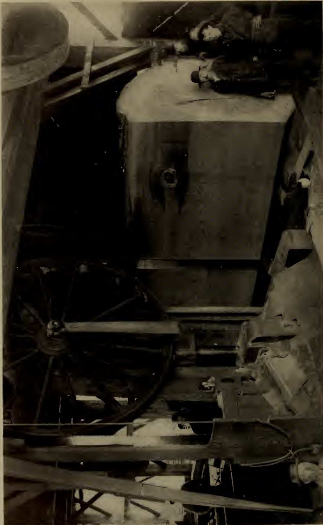
FIRST STEEL WHEEL on band saw head rig in redwoods. In the 90's, C. R. Johnson, founder of Union Lumber Company, braved ridicule in introducing band saws which first used wooden wheels. Arm at left controlled belt to wheel, was hinged to clear big redwood logs. (Photo Union Lumber Company Collection)
