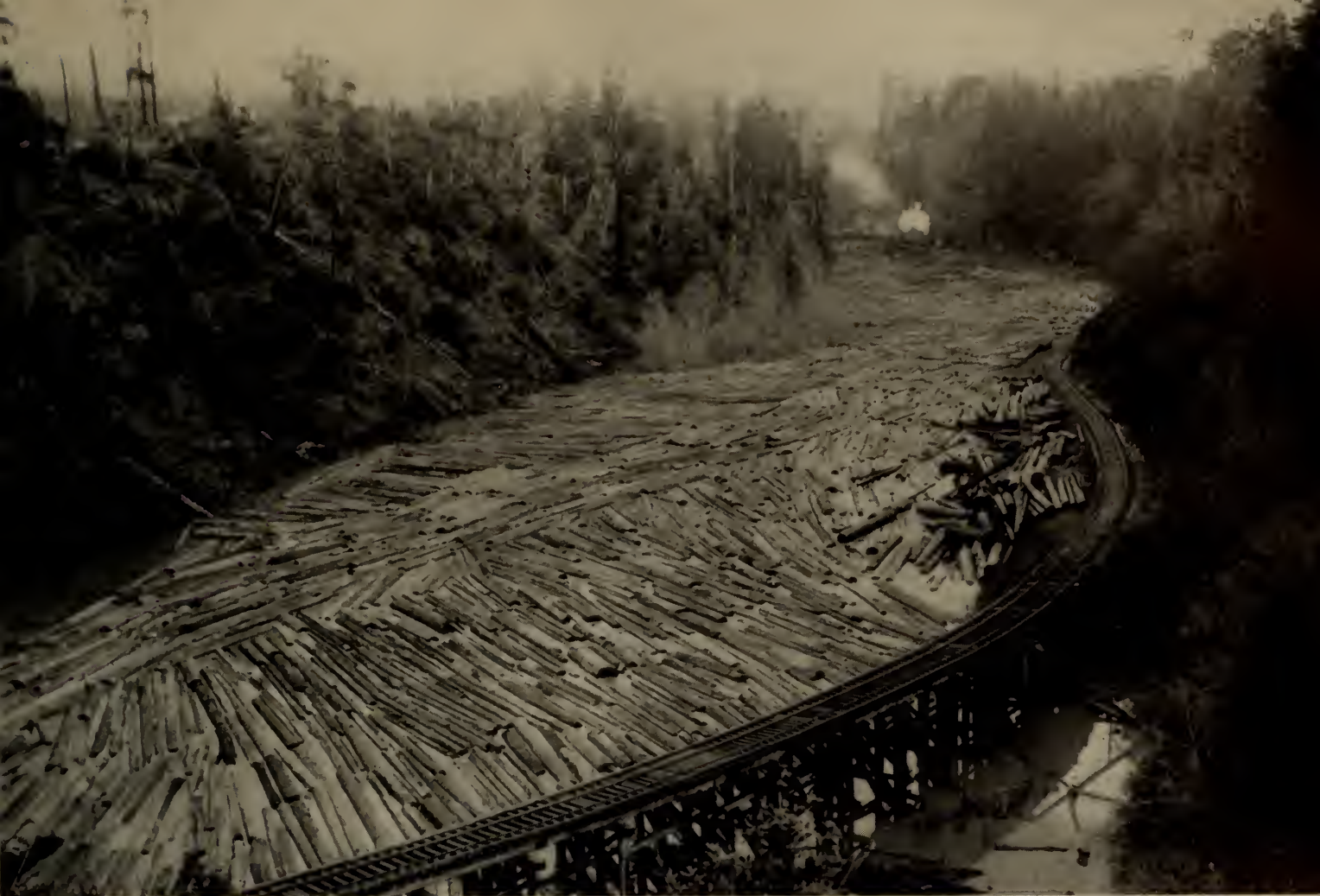
20 MILLION FEET of redwood logs in this Pudding Creek winter storage. From 1906 to 1916, Union Lumber Co. removed logs by incline and railroaded them one mile to mill at Fort Bragg. (Photo Union Lumber Company Collection)
