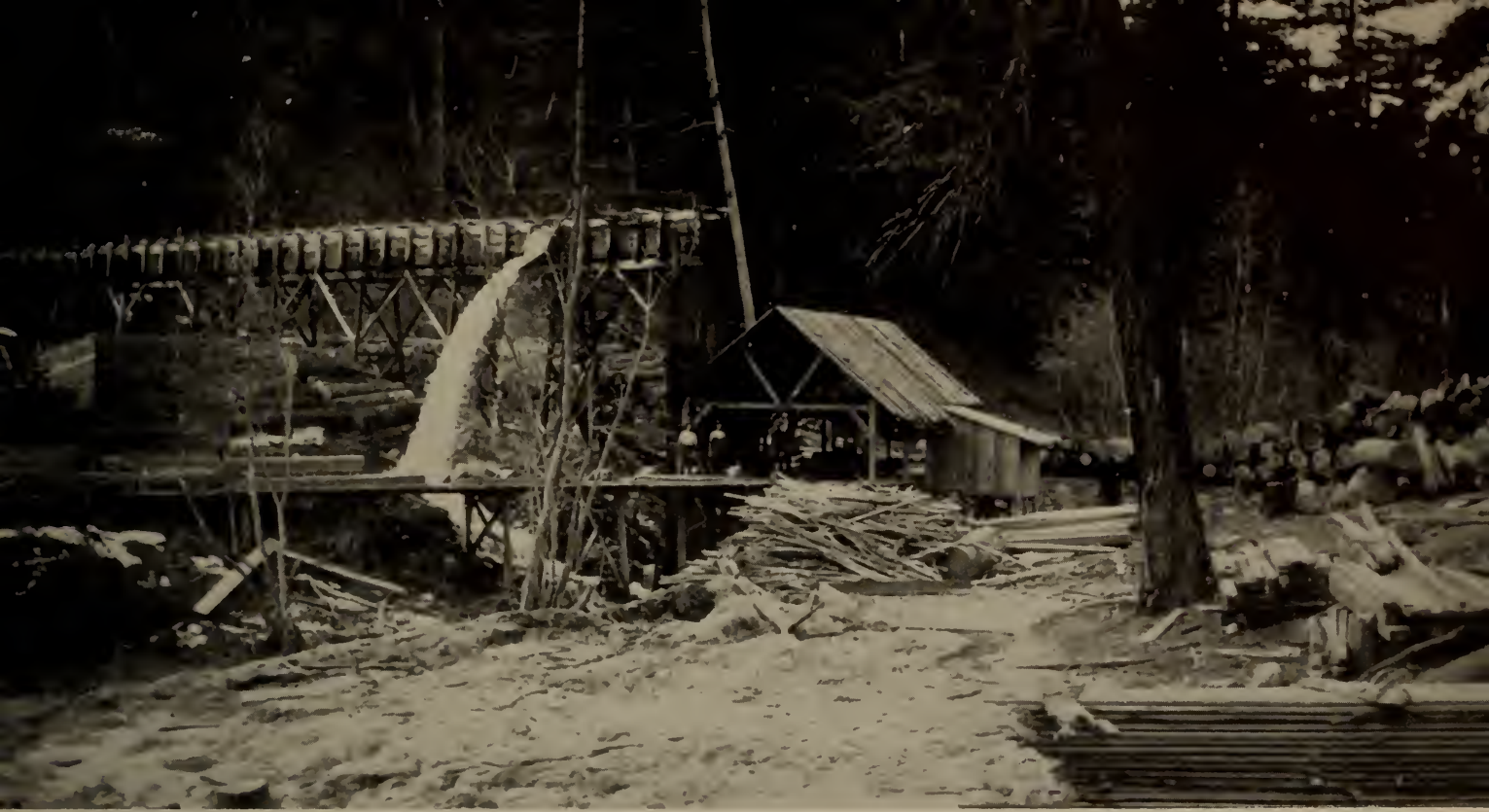
WATER POWER AT THE DALLES Manchester and Lester waterpower sawmill at Five Mile Creek, Oregon, about 1908. (Photo courtesy G. E. Manchester)
