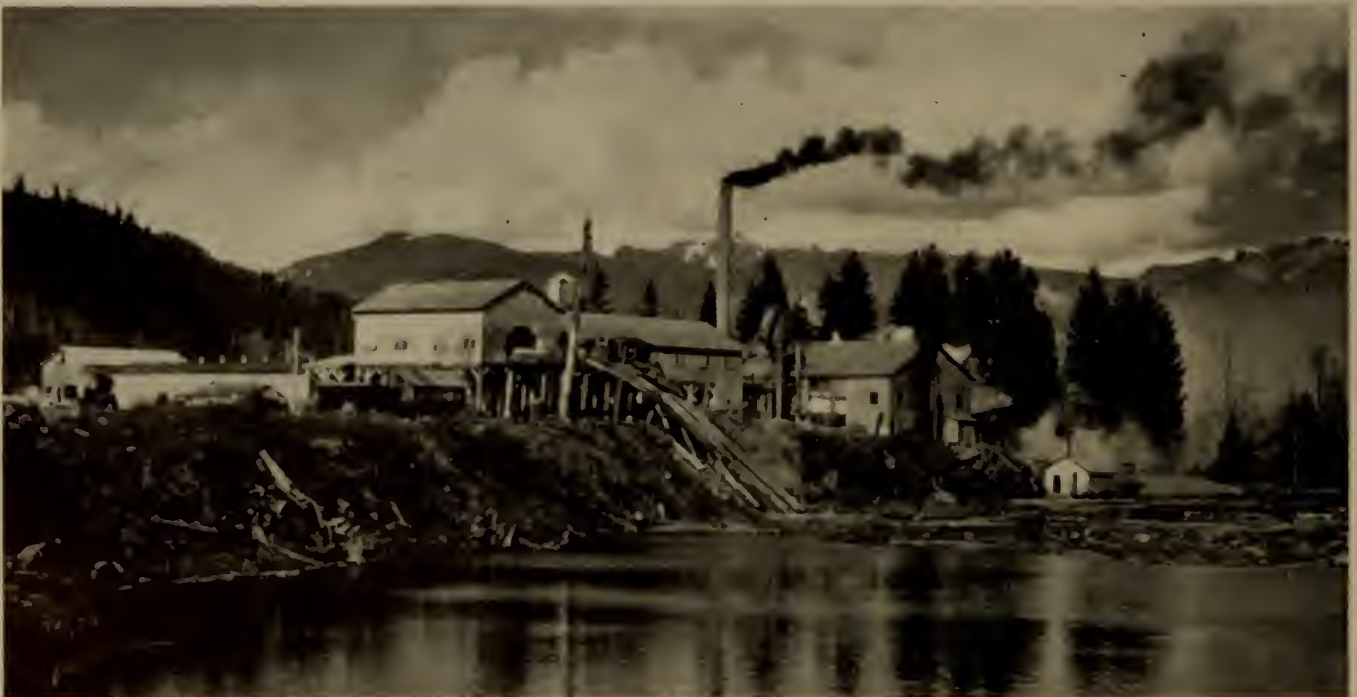
DARRINGTON MODERN Three Rivers Plywood and Timber Co. owned by E. E. and Roger A. Boyd, manufacturing on the scene made historic in highball logging days. (Photo courtesy E. E. Boyd)
